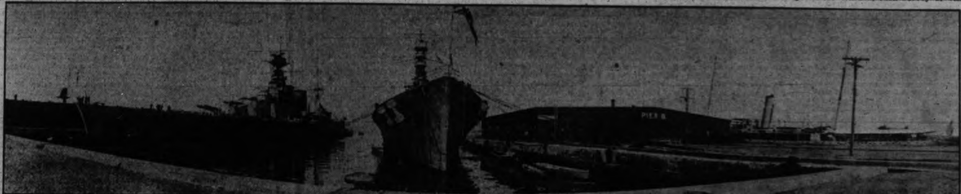
Some Idea of the Accommodation of the Outer Docks can be Gleaned from this—Two Great Battleships Docked and Room to Spare
